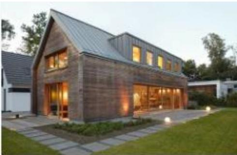
The roof was clad over an area of 180 m<sup>2</sup> with RHEINZINK-prePATINA blue-grey in the angled standing seam system, the timber façade is made of Douglas fir.
